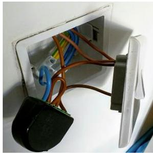
Figure 2: T-SW installation behind a wall switch
